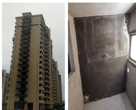
Figure 16: The Futian Cangjun building
